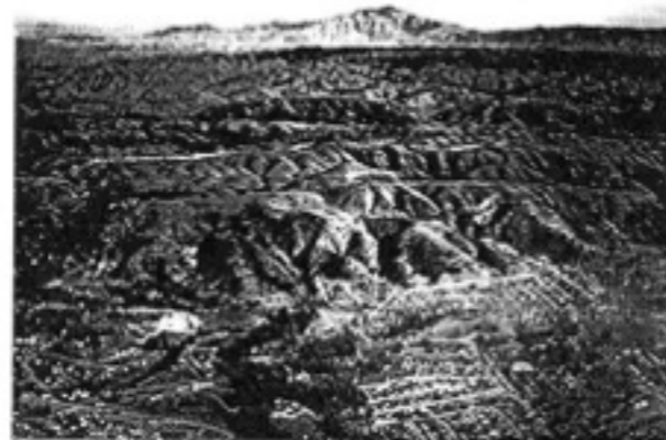
Overview of the changes in vegetation and structures in the East Bay Hills: 1934 Leona Heights, Oakland
