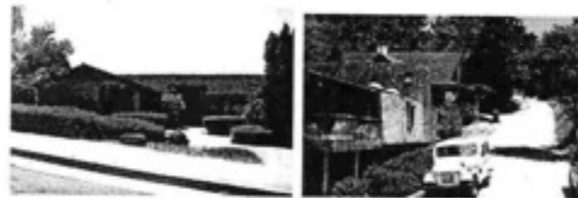
Structural hazards are evaluated based on the amount of wood roofs & wood siding/ decking in neighborhoods.
